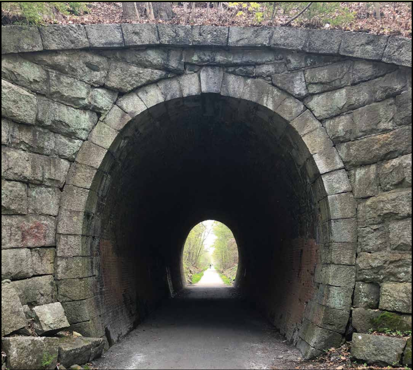
“Phipps Tunnel, Holliston”
