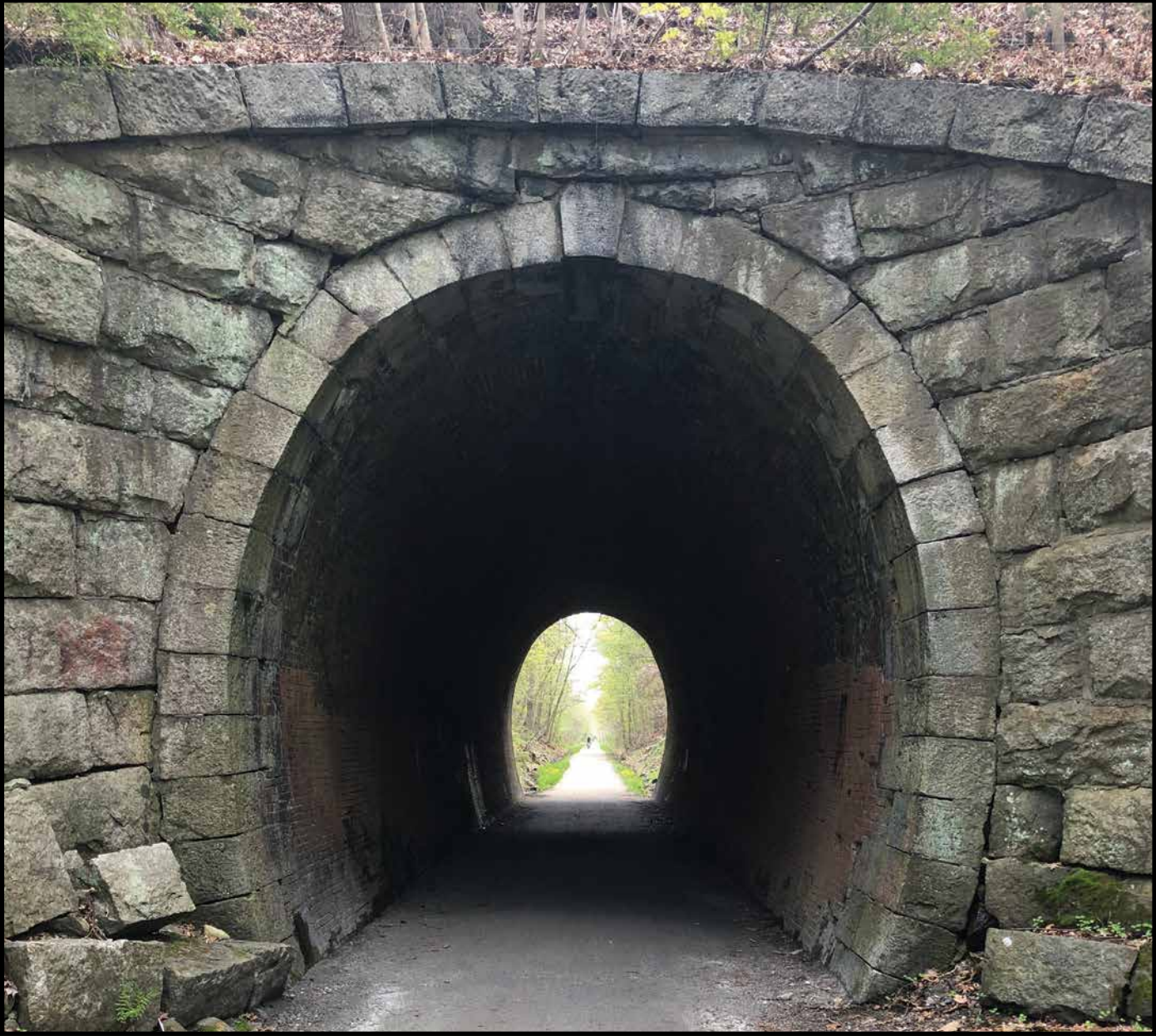
“Phipps Tunnel, Holliston”
